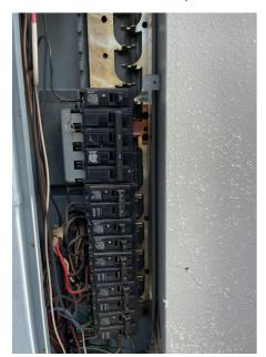
Wiring: Solid strand aluminum wiring present
