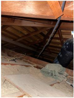
**Insulation: Type**Cellulose loose fill
